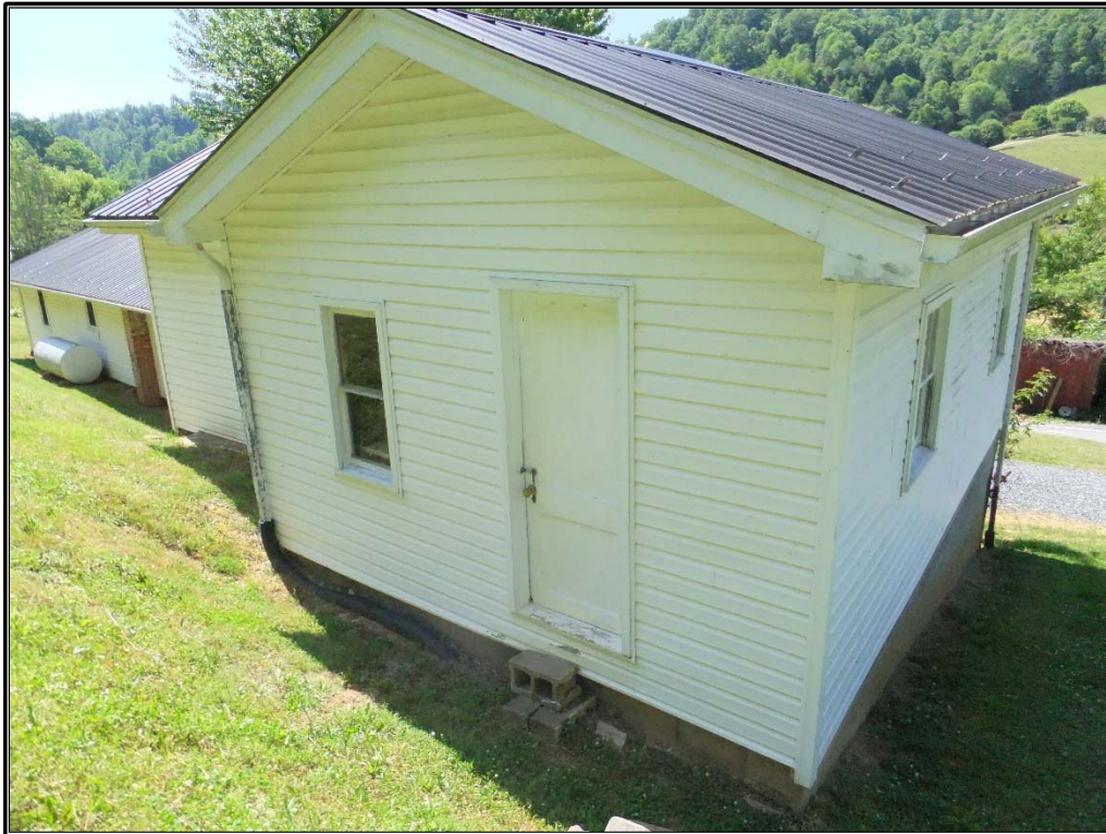
Figure 10. Rear of the garage associated with the J.W. Webb House (ML0128), facing northwest.
