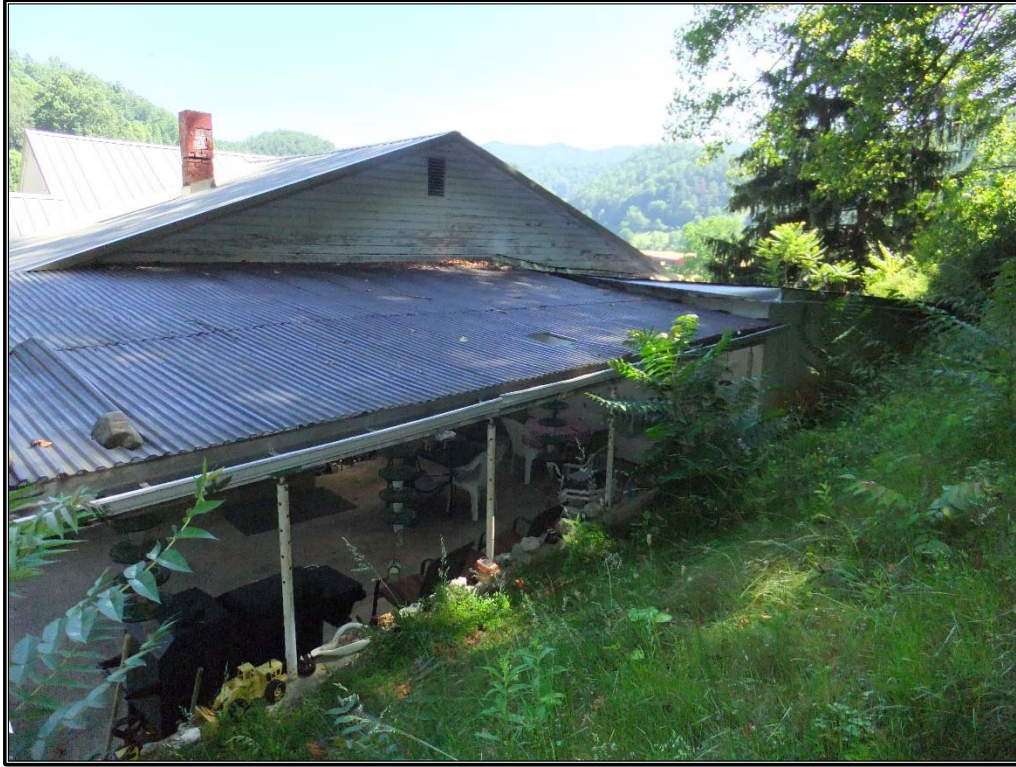
Figure 89. Exterior of the carport, facing northeast.
