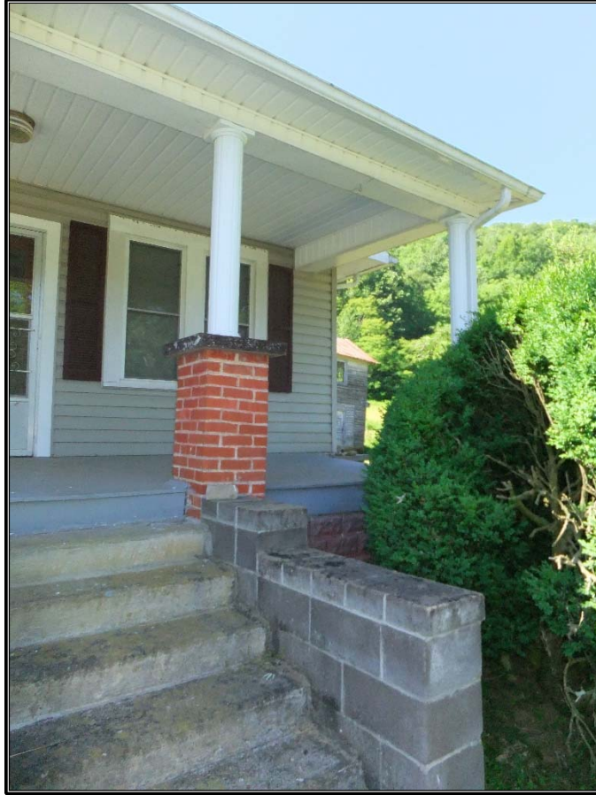
Figure 38. View of the porch details of the D.W. Tipton House (ML0129), facing southwest.
