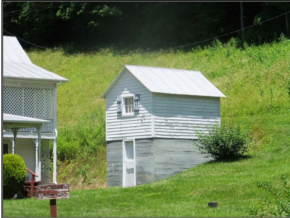
Figure 74. Detail of the cellar associated with the farmstead t 11842 NC 197, facing north.
