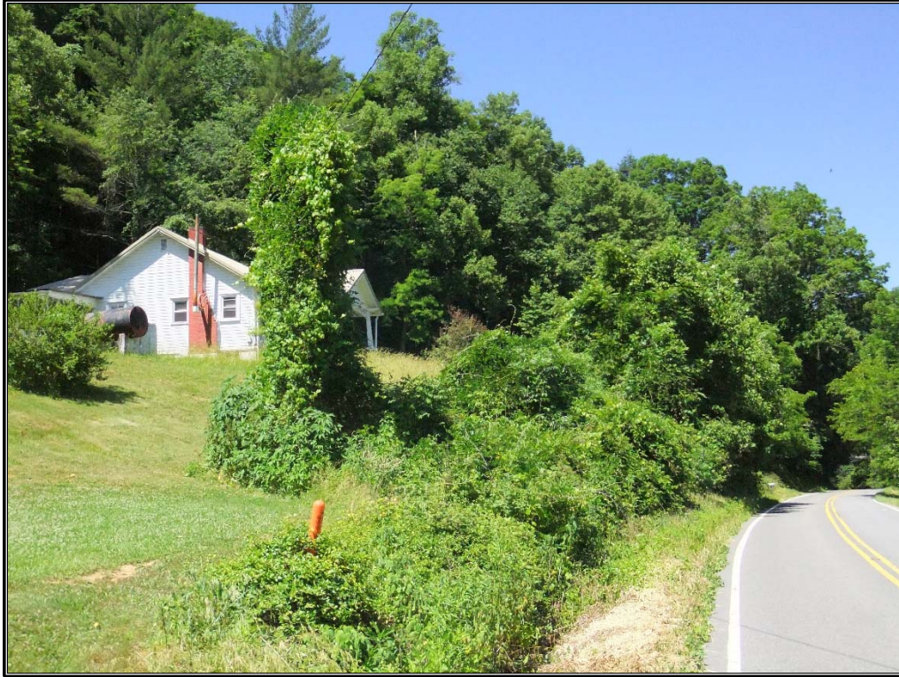
Figure 81. Overview of the Eston Pate House (ML0131) from NC 197 showing vegetative buffer, facing west-southwest.
