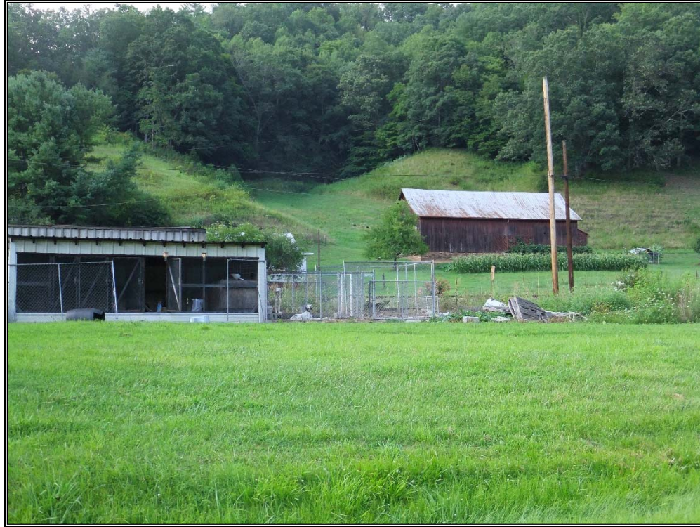
Figure 31. Overview of farm with barns along Hunt Dale Road (SR 1320) in the community of Hunt Dale in Mitchell County.
