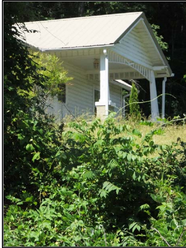
Figure 85. Detail of the porch of the Eston Pate House (ML0131), facing southwest.
