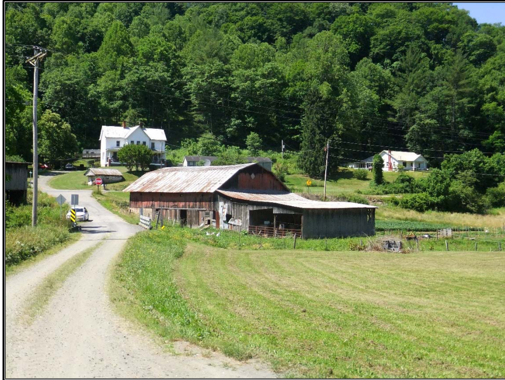
Figure 58. Overview of the house, barn, and outbuildings associated with the Whitson-Tipton Farmstead (ML0130) and Bridge No. 183 over Brummett Creek, facing south-southwest.
