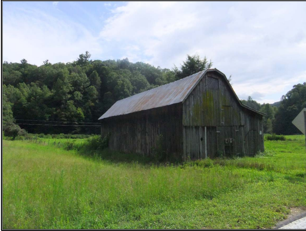
Figure 27. View of a gambrel-roof barn on NC 197 southeast of the community of Poplar in Mitchell County.
