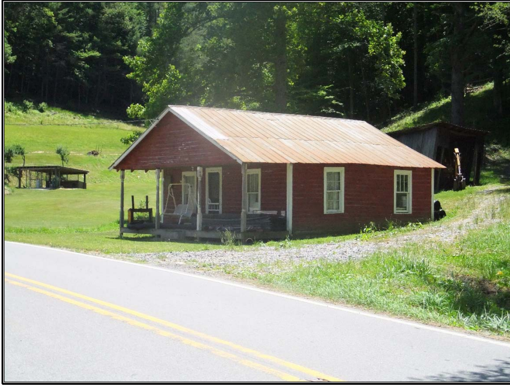
Figure 50. Comparable front-gable residence with drop siding on NC 197 in Tipton Hill, facing southwest.
