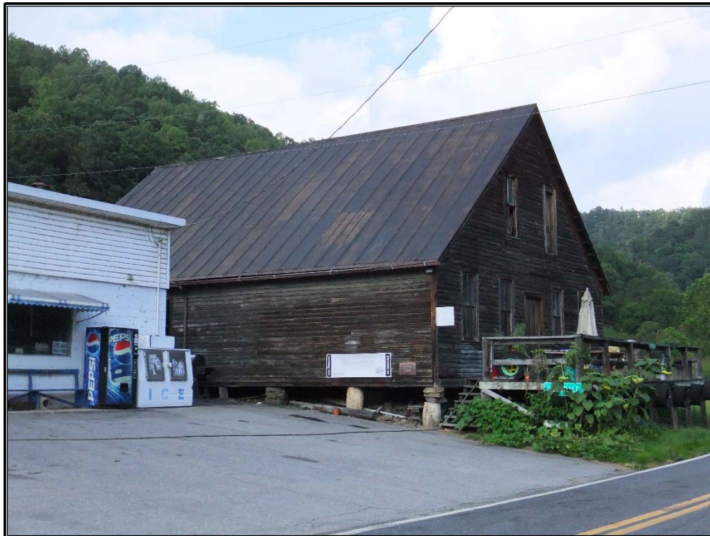
Figure 55. View of the early-twentieth-century front-gable Phin Peterson store on Hunt Dale Road in Hunt Dale, Mitchell County.
