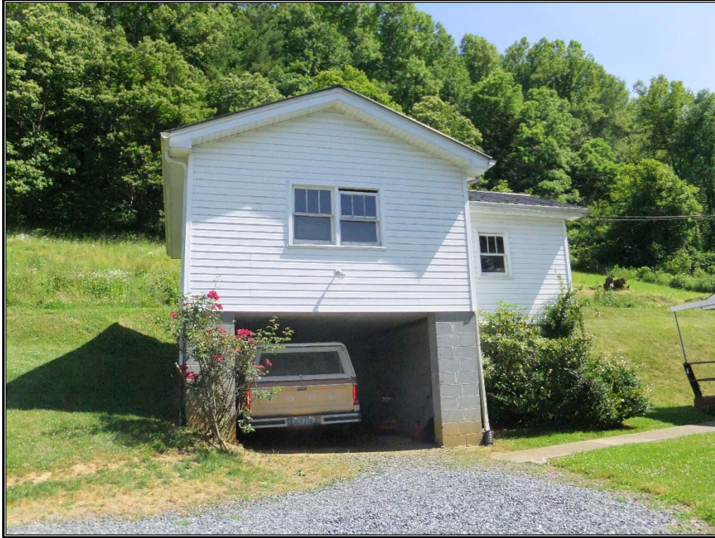
Figure 9. Façade of the garage associated with the J.W. Webb House (ML0128), facing south-southeast.
