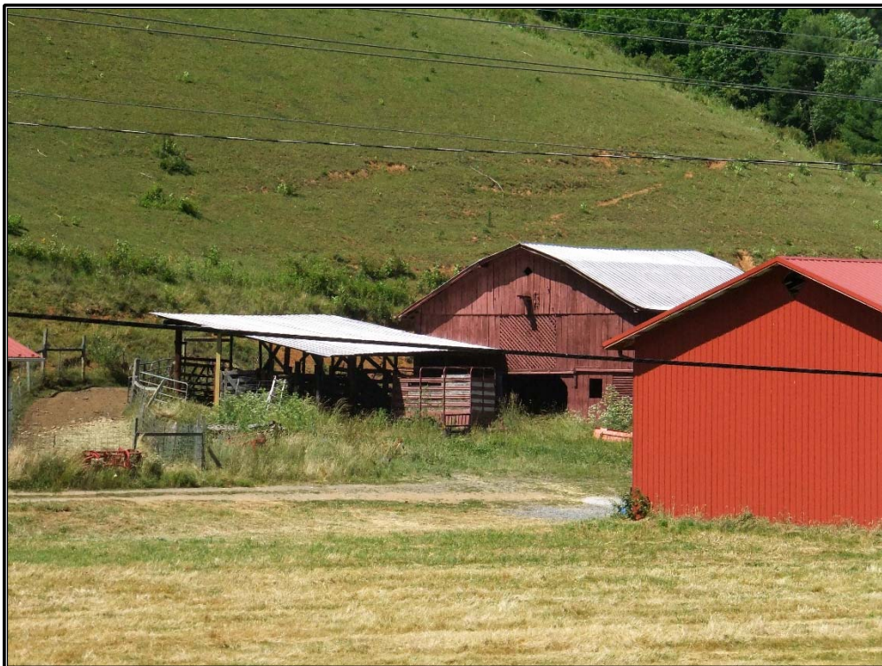
Figure 22. View of the façade and attached open shed of Historic Barn #2 on the J.W. Webb Farm (ML0127), facing northeast.
