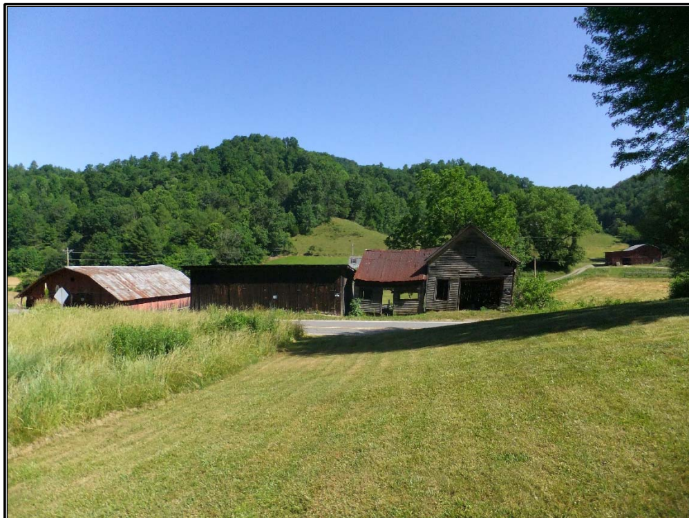
Figure 35. Overview of the shed and service station/store associated with the D.W. Tipton House (ML0129), facing north-northwest.
