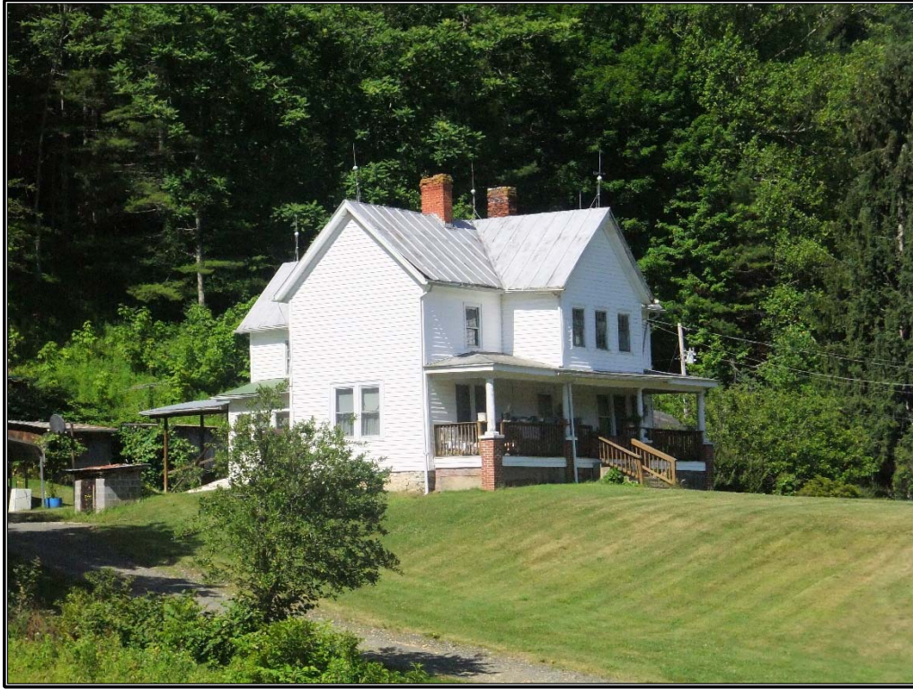
Figure 60. View of the façade and east elevations of the Whitson-Tipton Farmstead (ML0130), facing southwest.
