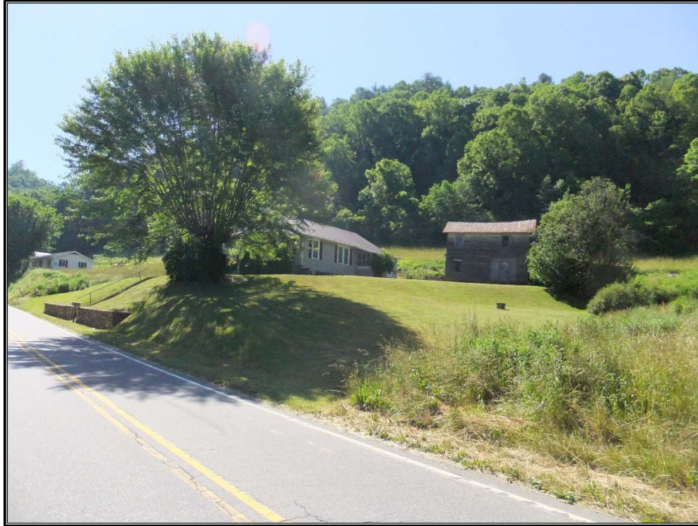
Figure 34. Overview of the house, nineteenth-century structure, and shed associated with the D.W. Tipton House (ML0129), facing east.
