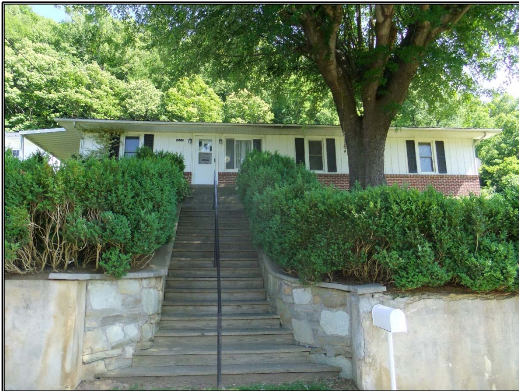
Figure 4. View of the retaining wall and steps that connect the J.W. Webb House (ML0128) from NC 197, facing south-southwest.
