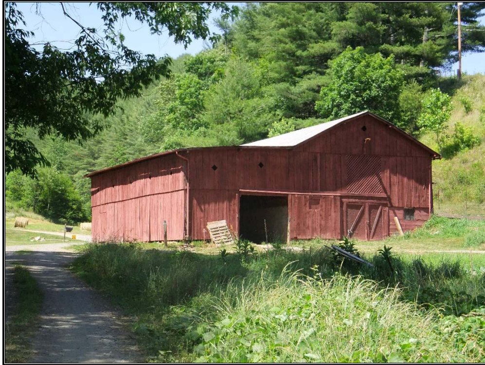
Figure 19. View of the circa 1900 Historic Barn #1 located east of Miller Road, part of the J.W. Webb Farm (ML0127), facing north-northeast.
