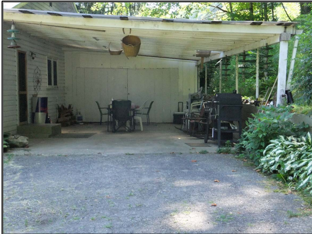
Figure 88. Interior view of the carport on the rear of the Eston Pate House (ML0131), facing east.
