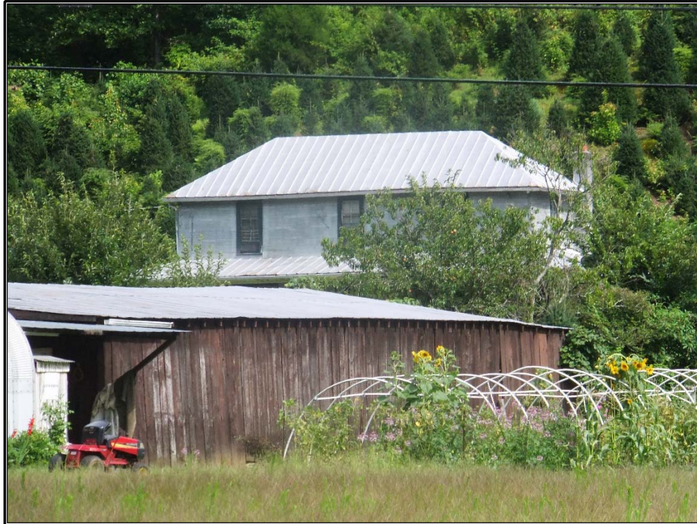
Figure 78. Agricultural outbuildings associated with a farmstead on Pigeon Roost Road (SR 1349), facing southeast.
