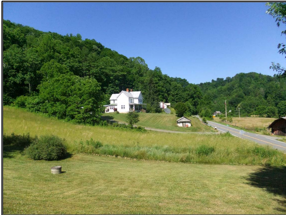
Figure 59. Overview of the Whitson-Tipton Farmstead (ML0130) and outbuildings, facing southwest.
