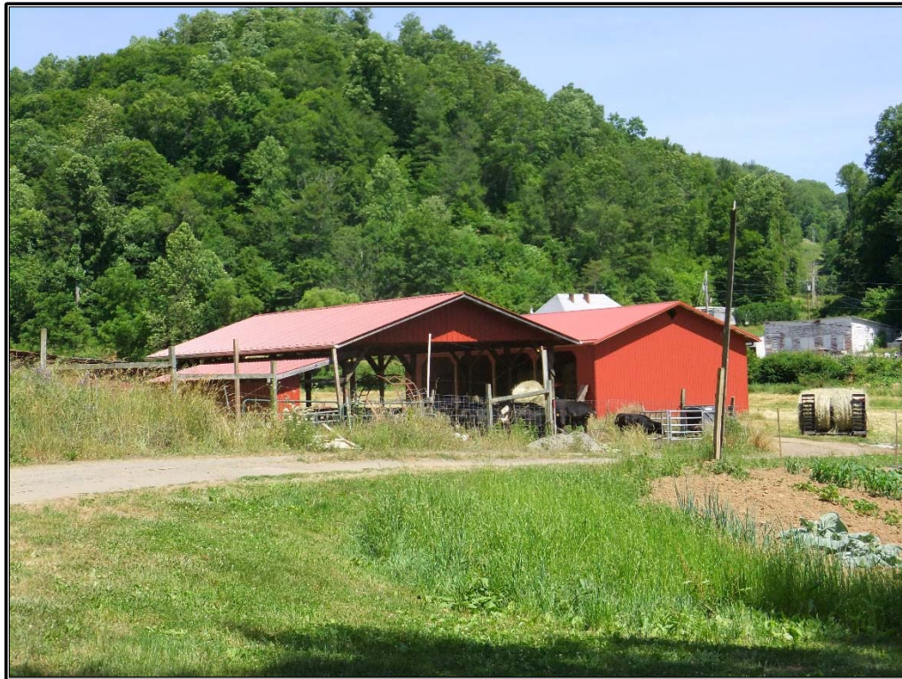
Figure 24. View of Modern Pole Barns #1 and #2 associated with the J.W. Webb Farm (ML0127), facing east.
