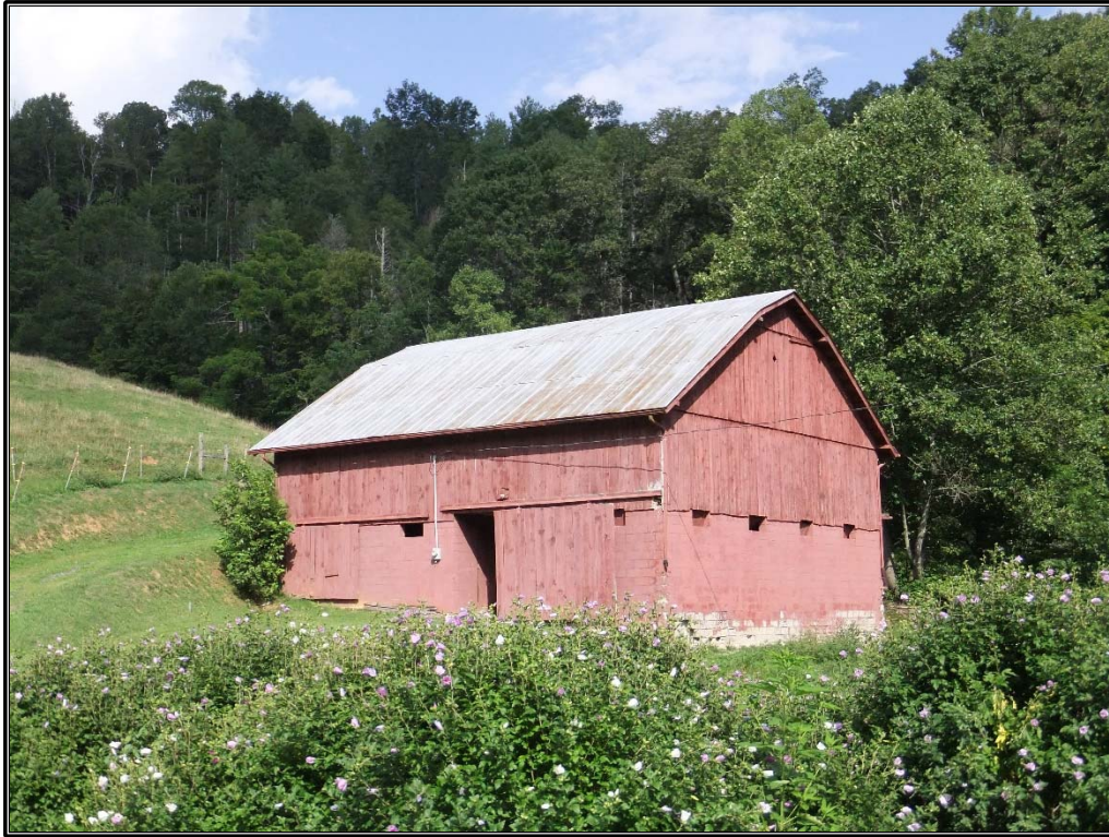
Figure 28. View of a gambrel-roof barn on NC 197 northwest of the community of Relief in Mitchell County.
