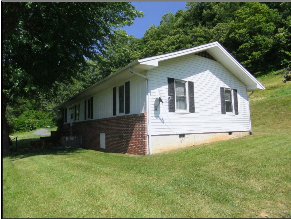
Figure 8. Façade and side, or southwest, elevation of the J.W. Webb House (ML0128), facing east.
