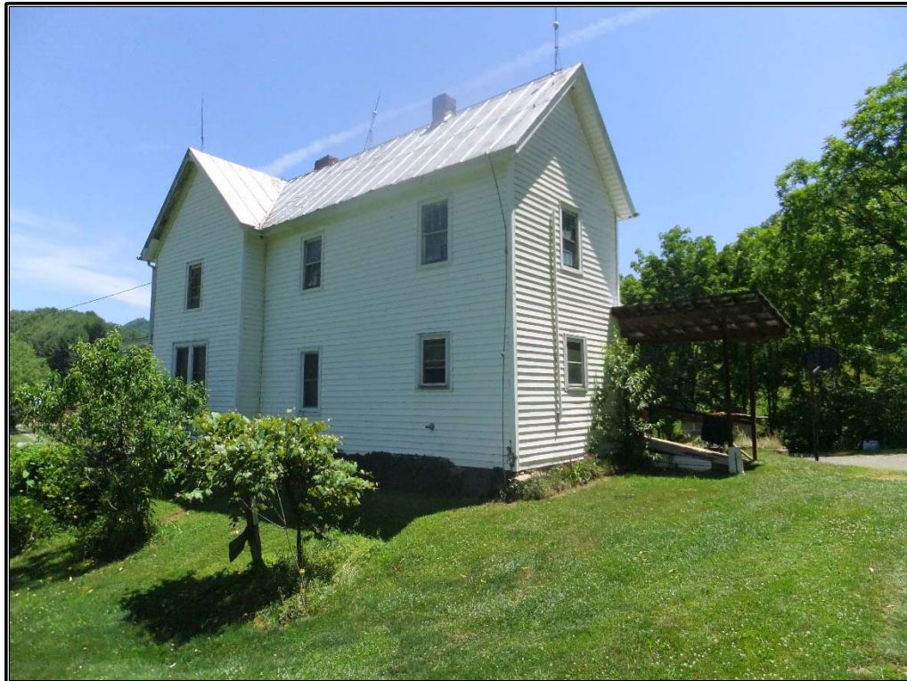
Figure 63. Rear and west elevation of the Whitson-Tipton Farmstead (ML0130), facing northeast.
