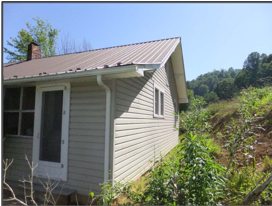
Figure 41. Rear elevation of the D.W. Tipton House (ML0129), facing north-northeast.
